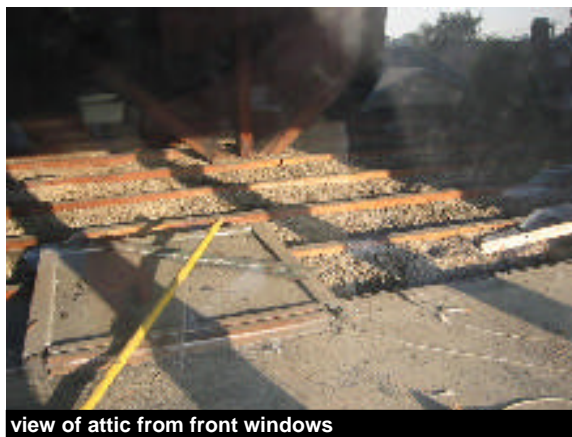
view of attic from front windows
