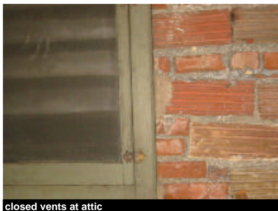
closed vents at attic
